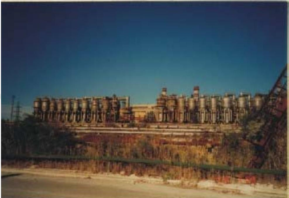
Figure 2. Evaporators for the nuclear desalination plant (Liquid Metal-cooled Fast Breeder Reactor (LMFBR) connecting an Multi-Effect Distillation (MED) Facility) in Aktau, Kazakhstan.
