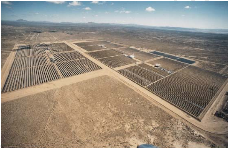
Figure 2. The five 30 MW e parabolic trough power plants SEGS III to VII at Kramer Junction in California (USA). (Source: Pilsolar)
